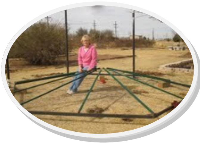
Linda Jarvis sits on the roof of the new Education Garden gazebo before installation.
